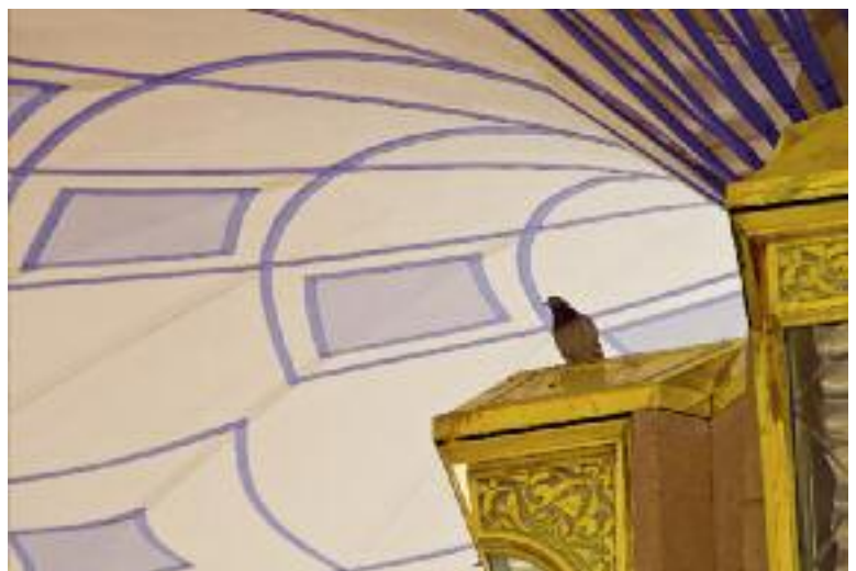
Applications made from blue PTFE-ribbons form oriental patterns on the underside of the umbrellas.
