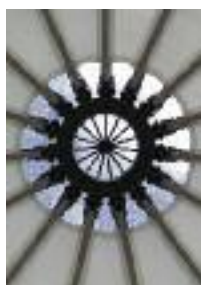
Title page Detail of the retractable membrane roof at the Kufstein Fortress Arena with SEFAR® Architecture TENARA® fabric.
